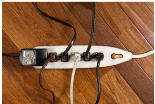
Don't overload extension cords or wall sockets.
